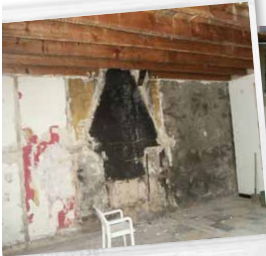
Before the renovation
